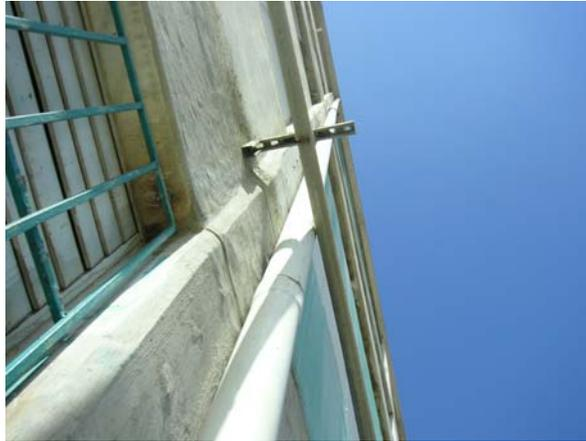
Photograph #2 15 meter 4 inch pipe used as solar chimney
