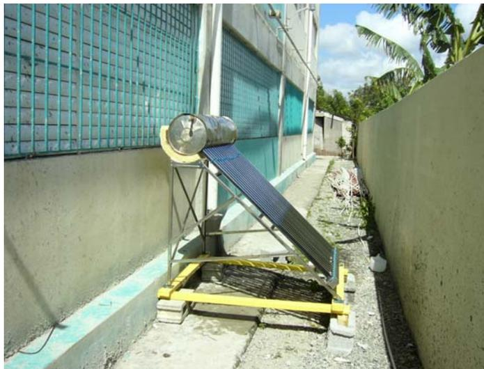
Photograph #1. Concentric Vacuum Tubes Solar Collector.
