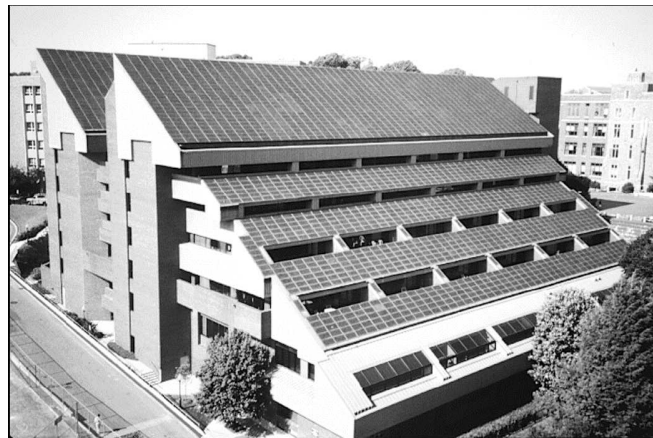
Figure 10: The Georgetown university in Washington DC designed with PV roof (Courtesy: Solar design associates, Inc.)
