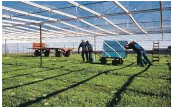
Figure 17: Roof of the collector in Manzanares (Spain)
