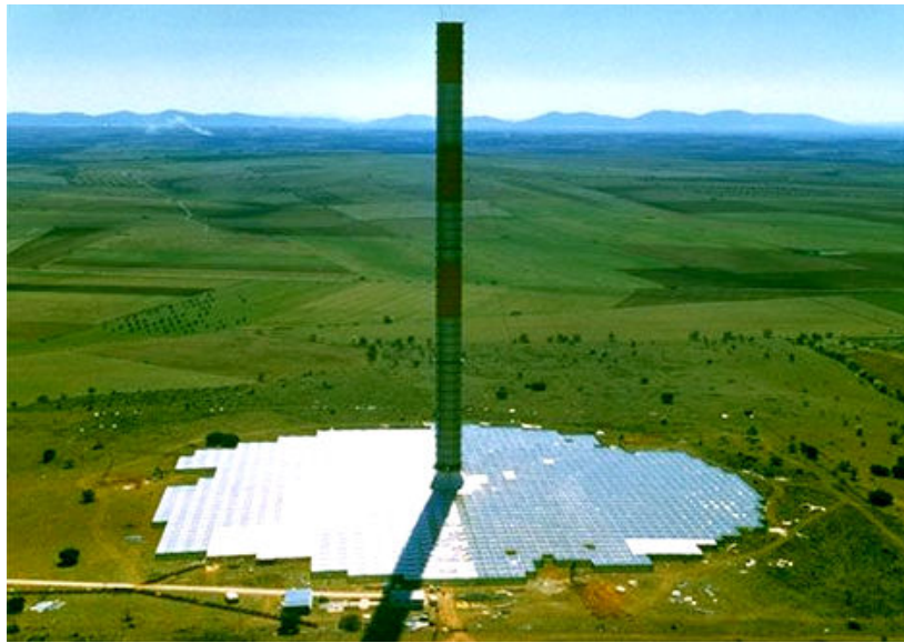
Figure 6 50 kW Solar chimney pilot project , Manzanares, Spain
