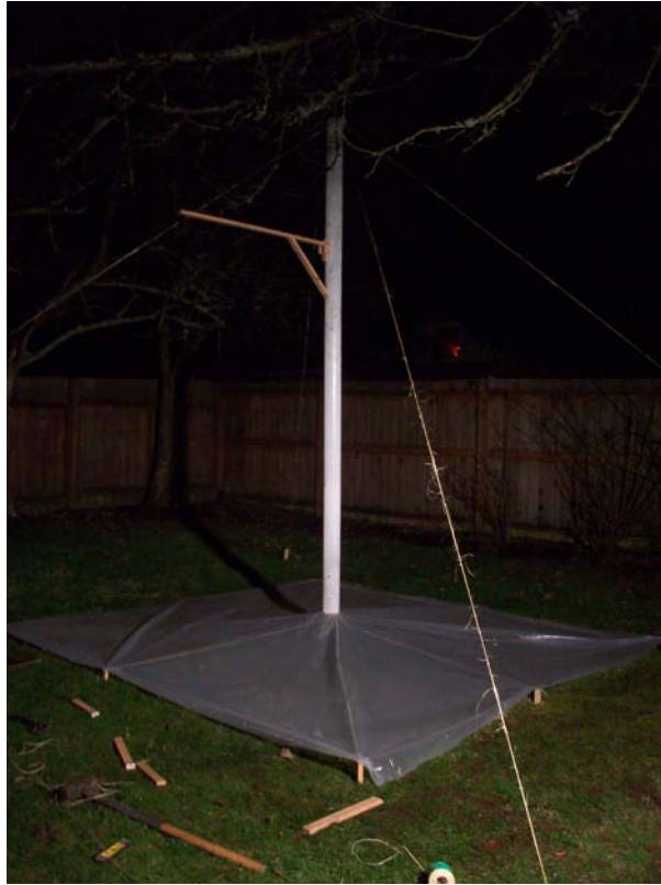
Figure 2 Photo taken of actual chimney
